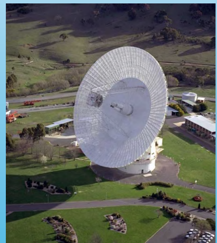
The antenna "listens" for signals from space. It has a diameter of 70 meters and is located in Australia. Photo: nasa.gov
